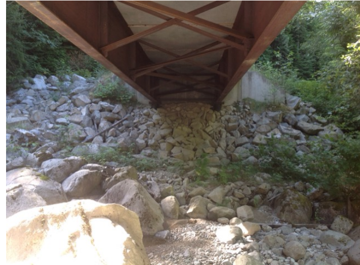
Left Bank Abutment when facing downstream
