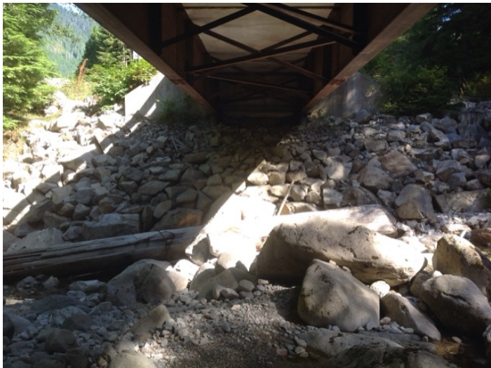
Right Bank Abutment when facing downstream
